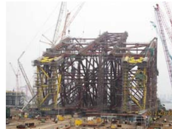
Current status of jacket fabrication
