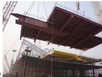
Topsides fabrication is proceeding on schedule
