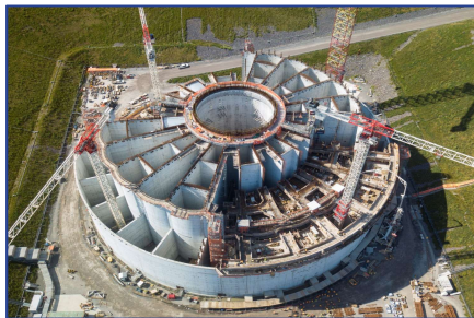
West White Rose Project Quadrants Completed
