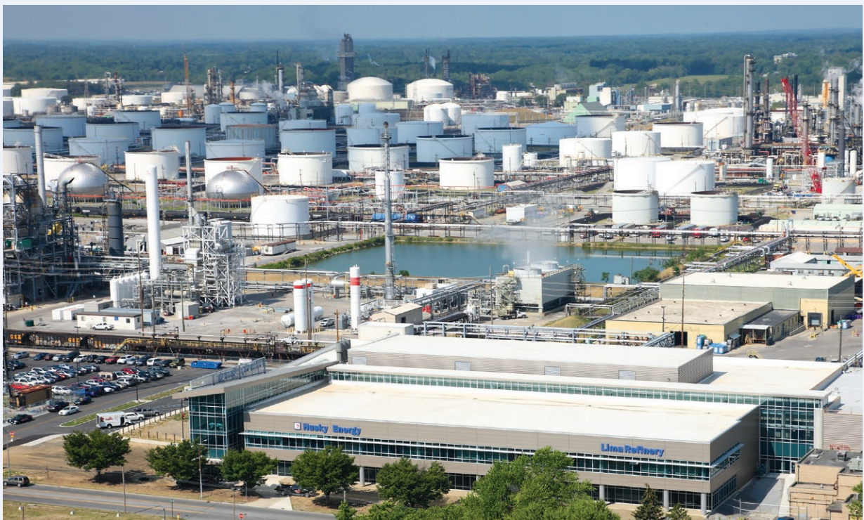
The crude oil flexibility project at the Lima Refinery will increase heavy oil processing capacity to 40,000 bbls/day by the end of 2019.
